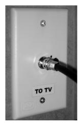
To use the TV antenna, turn "ON" the switch located on the TV jack. A light will show on the indicating the antenna booster is powered. There will be a small continual 12-volt current drain as long as the switch is on. Turning the switch "OFF" changes the TV jack from antenna operation to park cable and ceases the current draw.
