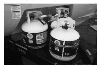
Dual propane tanks are equipped with a two-stage automatic changeover regulator, which transfers propane demand automatically to the second tank when the first tank becomes empty.
