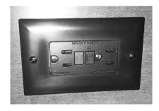
A Ground Fault Circuit Interrupter (GFCI) protects the bathroom, galley, and patio 120-volt receptacles. This device is intended to protect you against the hazards of line to ground electric faults and electrical leakage shocks possible when using appliances in damp areas.
